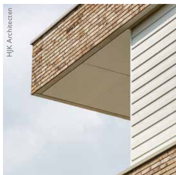
Buitenplafond in Cedral Board
